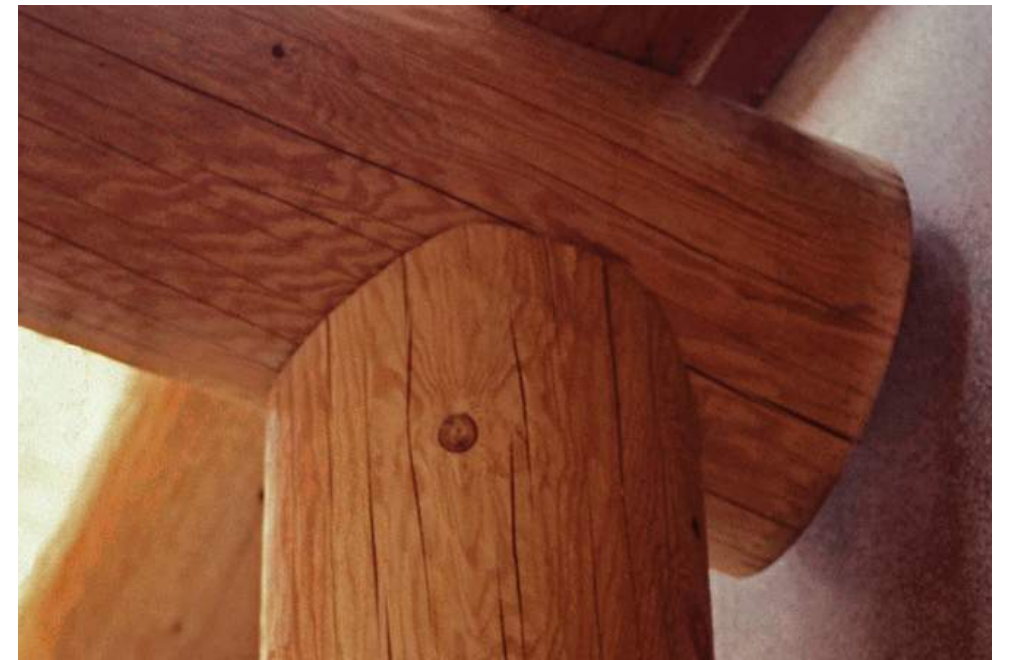
EXPOSED LOG/TIMBER CONSTRUCTION
