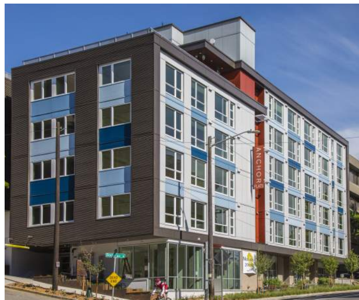
ANCHOR FLATS | SEATTLE, WA
